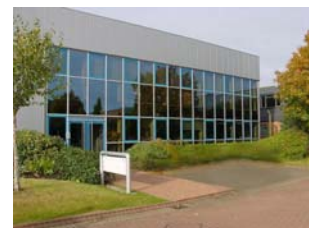
OpTek Systems HQ, Abingdon, UK
